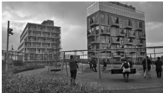
写真-6 Parkinghouse Luders (上：外観，下：屋上部)
